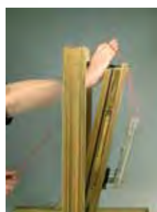
Open the window with the guide wire
